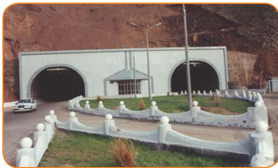
74-rasm. Qamchiq dovonidagi tunnel.
